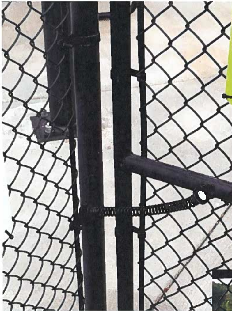
Metro Station Dog Park – Installed self-closing gate springs.
