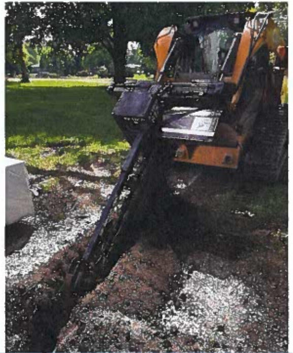
Round Barn – Repairing internet by dug/trenched to run new internet cable.
