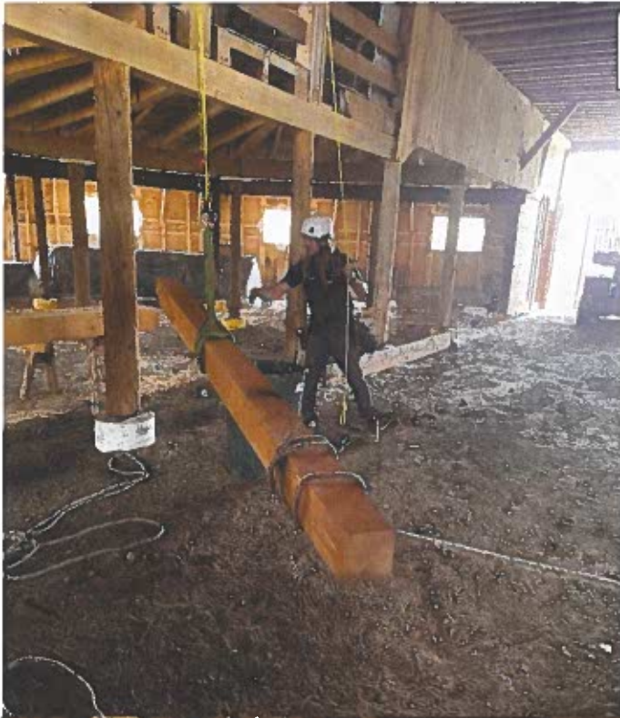
Round Barn – Hoisting large timbers inside roof of barn
