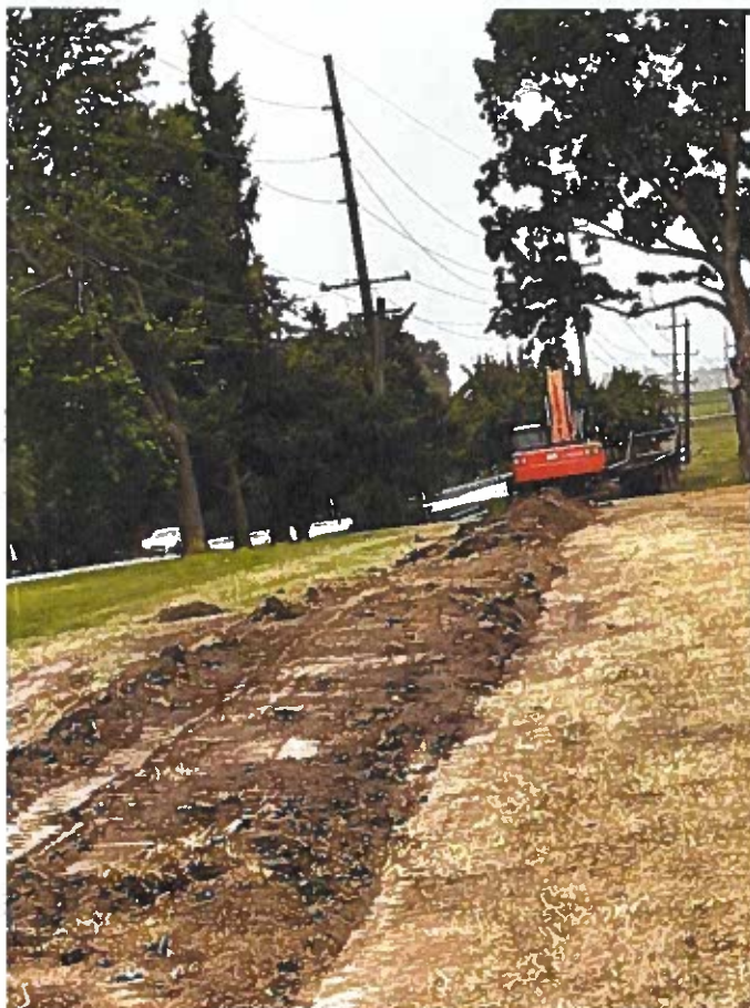
Round Barn – Installation of water main to barn.
