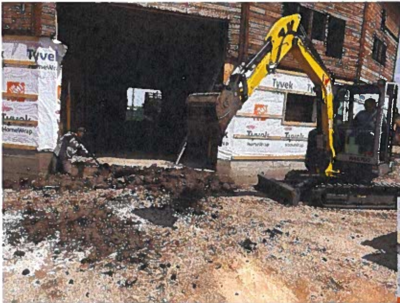
Round Barn – Installation of drainage pipe around barn and to Blacksmith Building .
