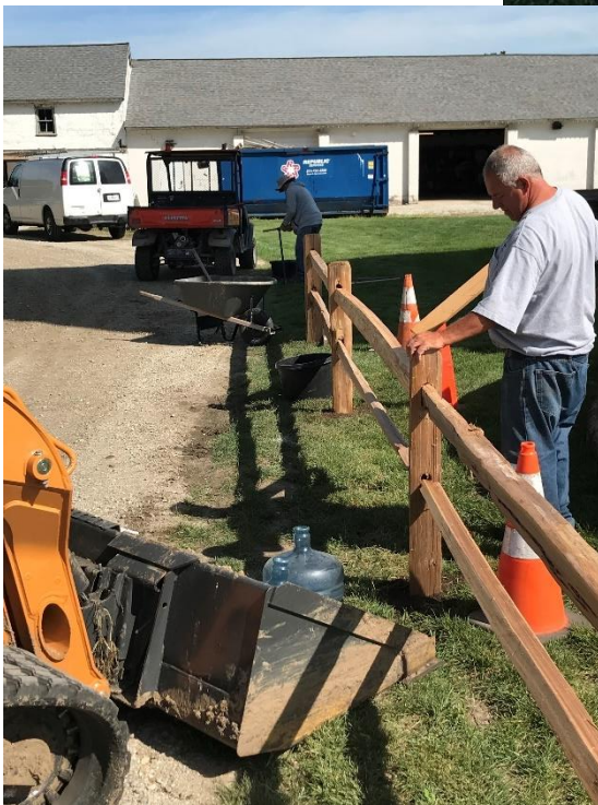
Round Barn – Installation of cedar split rail fence.
