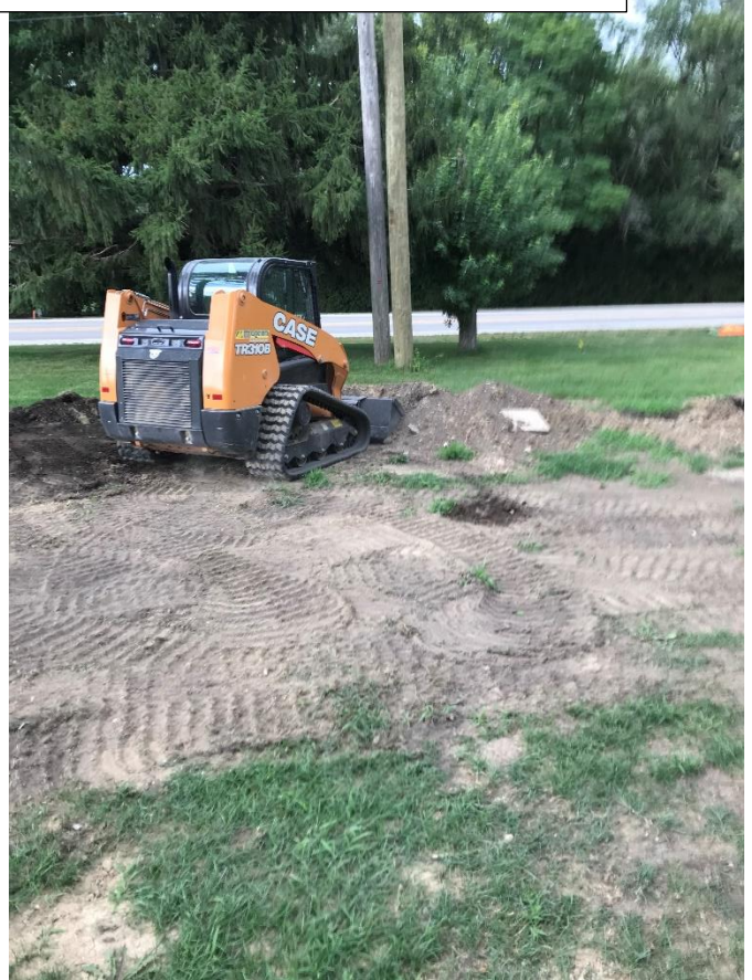
Round Barn – Graded, seeded and blanketed North entrance following water main installation.
