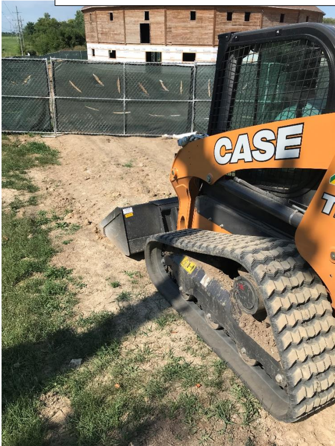
Round Barn – Graded, seeded and blanketed North entrance following water main installation.
