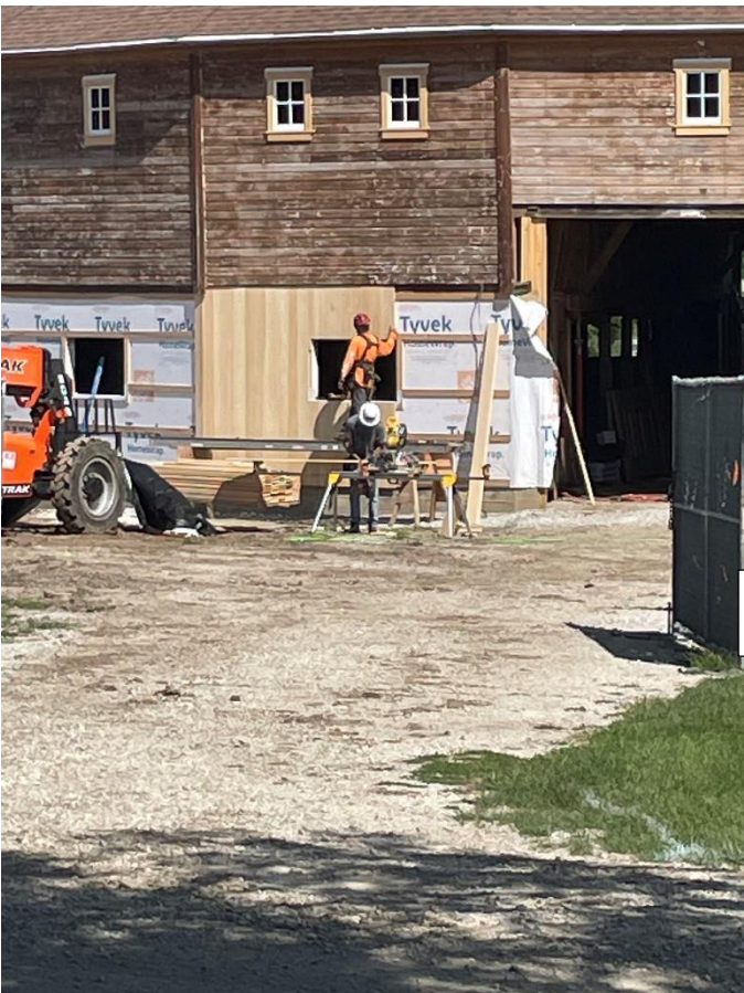
Round Barn – Installation of windows and wood siding.
