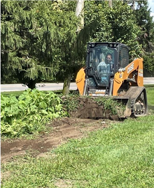
Round Barn – Grading front of property from water main installation.
